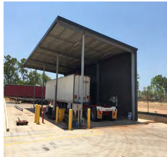
Source: Northline Plate 3-14 Example of vehicle wash down facility
