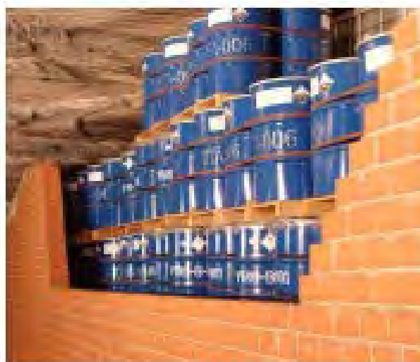
Plate 3-7 Example of simple single-skin wall seal in
