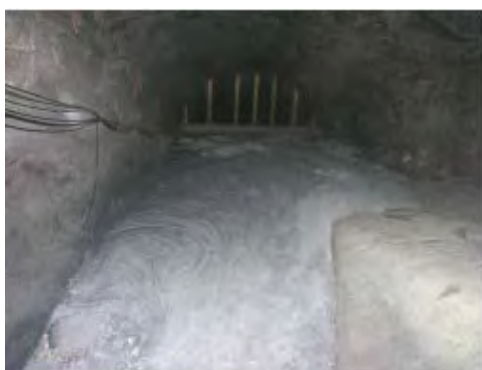
Plate 3-9 Typical underground hydraulic backfill
