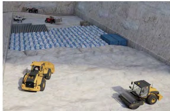
Open cut kaolin mine creates the voids (left). The voids are used for the safe and secure storage of waste in sealed containers (right).
